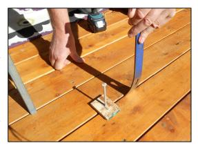
For the last step, go back and pre-drill two holes in all deck boards for each joist. Then place a screw in each hole down into the joist below to securely fasten the deck down.
