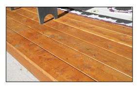
Juniper decking can be installed 16" or 24" on center. The deck shown here has been installed 24" on center.
