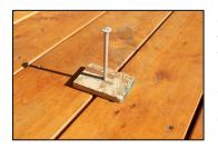
**4. Make your plan:** Walt suggests laying all the boards out, then securing them with one screw at each end and one in the middle prior to fully installing the deck. This way the pattern and spacing can be worked out and any adjustments made more easily than when each piece has been fully secured to all the joists below. Walt uses home-made spacers (see photo at left) to line the boards up at the right distance.
